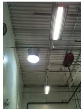
*Sun light tubes on left and smart lighting system on right, which adjusts wattage depending on light level and motion detection.*
